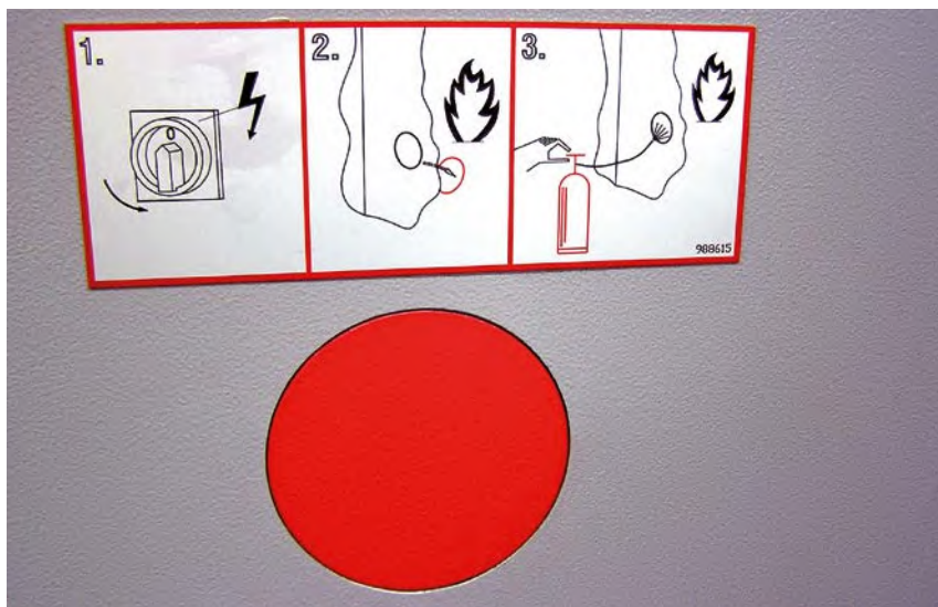
Figure 49 Extinguishing hole with marking and information
