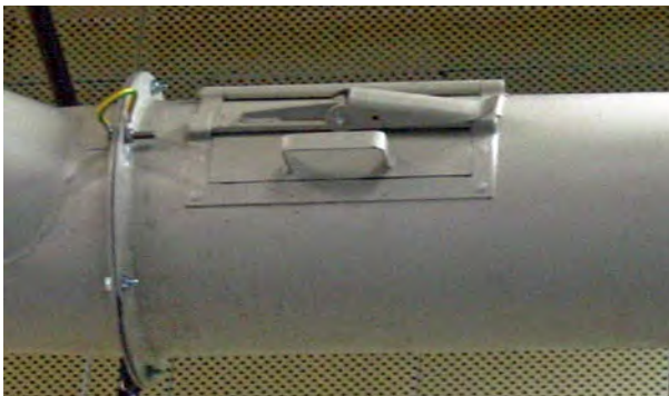
Figure 39 Inspection holes 2
