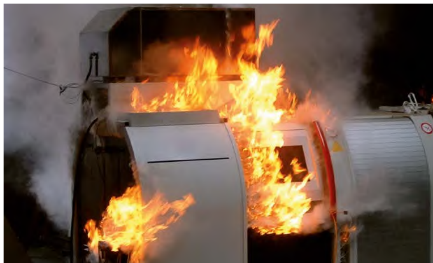
Figure 9 ... with subsequent fire
