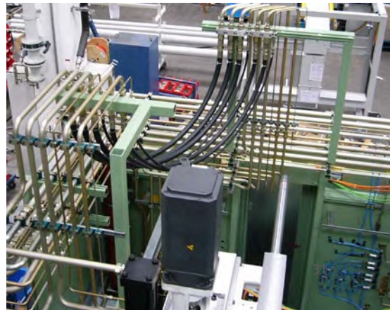
Fig. 11 Pipeline routing in a large machine
