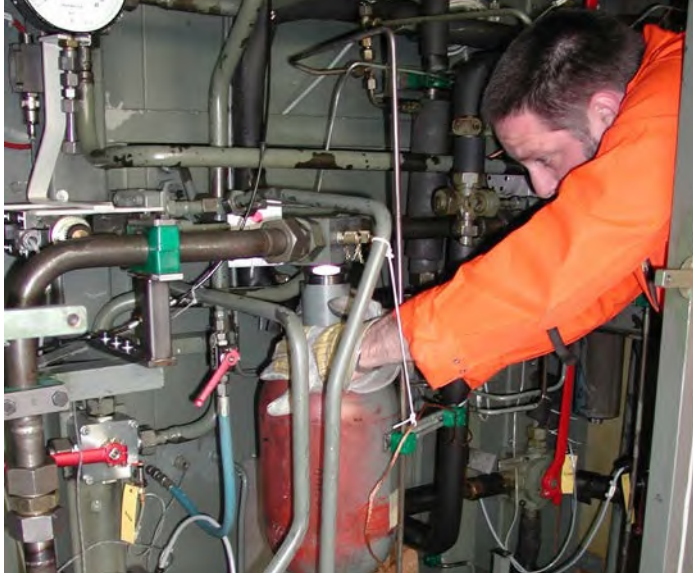
Fig. 1 Maintenance technician during maintenance work
