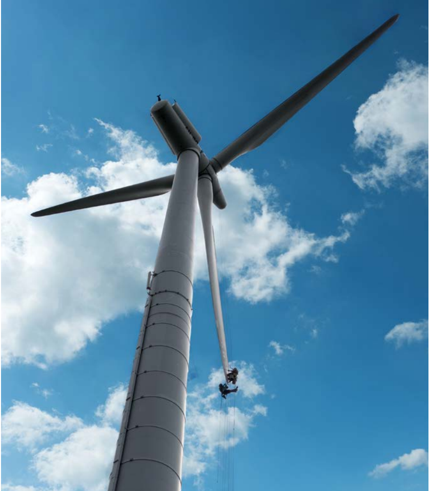
Abb. 43 Reparaturteam am Rotorblatt
