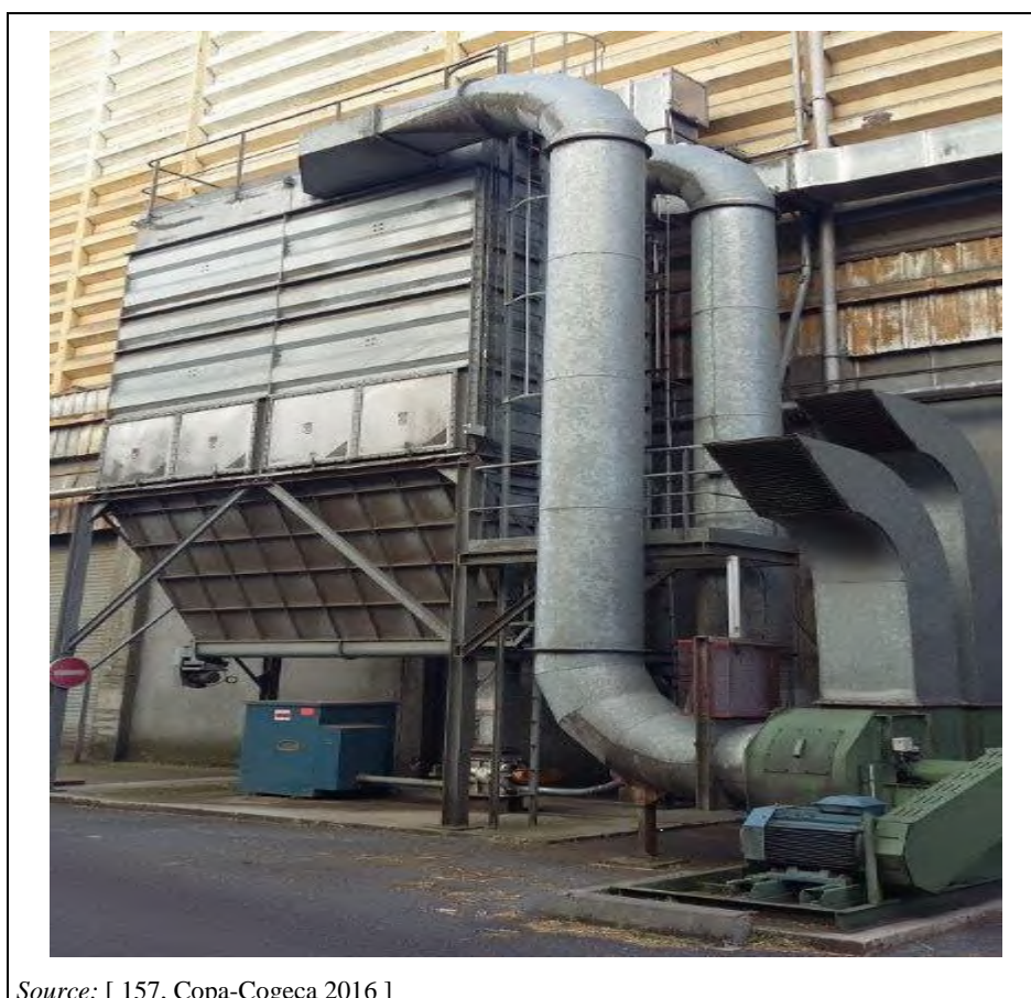
Figure 2.43: Picture of an industrial bag filter
