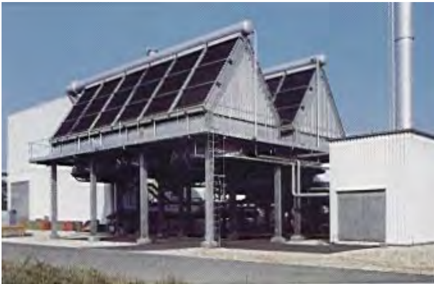
Figure 2.15: Example of an air-cooled condenser for condensation of turbine exhaust steam [tm111, BDAG, 1996]
