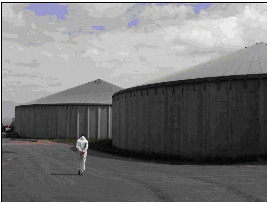
Figure 4.77: Rigid cover for slurry storage, with conical shape
