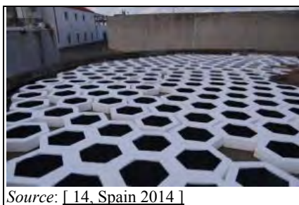
Figure 4.78: Geometrical plastic tiles in a slurry tank
