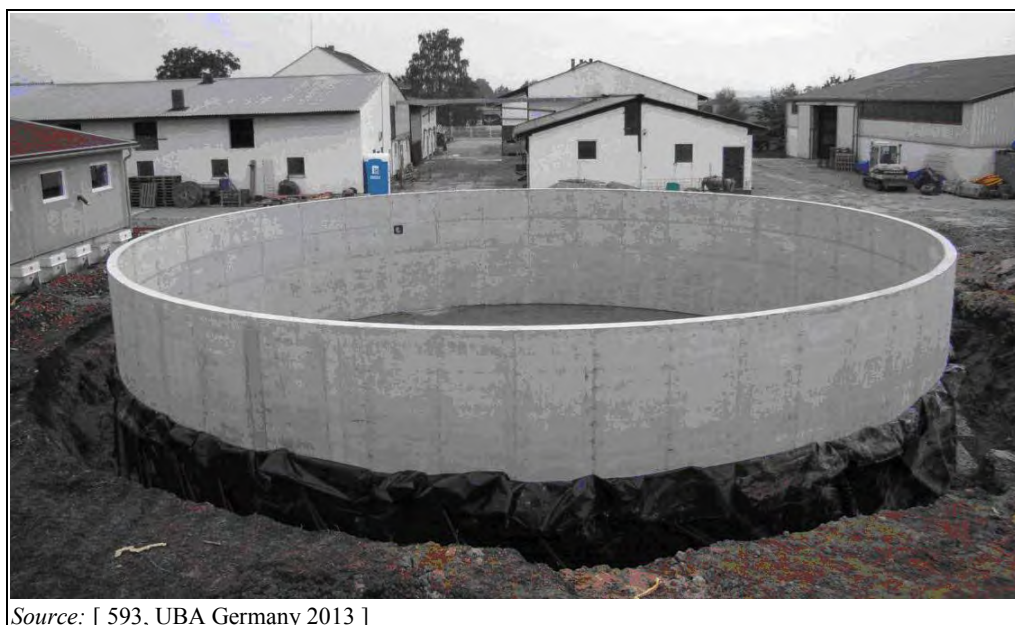
Figure 4.79: Underground slurry tank with liquid-tight geomembrane
