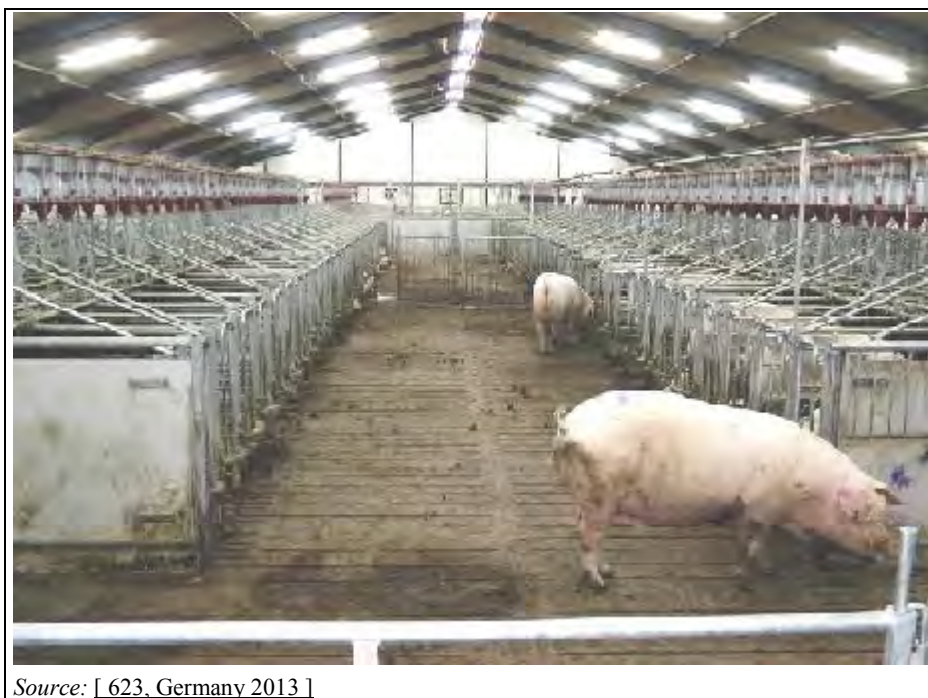
Figure 6.4: Gestating sow room of the near-zero-emission pig housing system showing the 'roof-ceiling' construction principle
