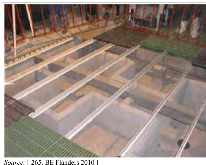
Figure 4.48: Shallow slurry pits separating manure and water channels during construction
