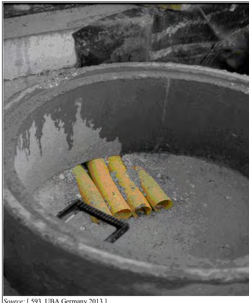
Figure 4.80: Inspection shaft for area drainage pipes from a slurry store
