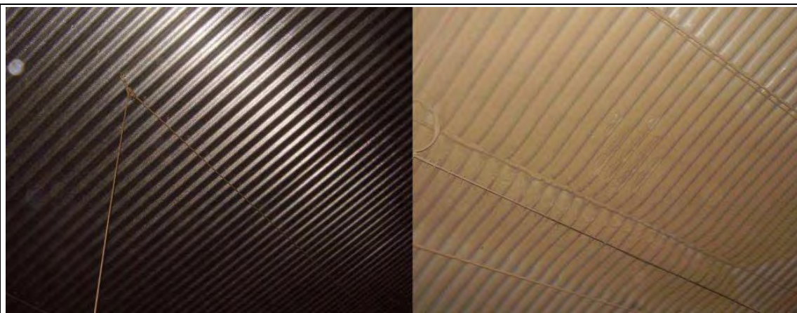
Figure 4.67: Effect of dust attraction caused by ionisation on the roof of a poultry shed
