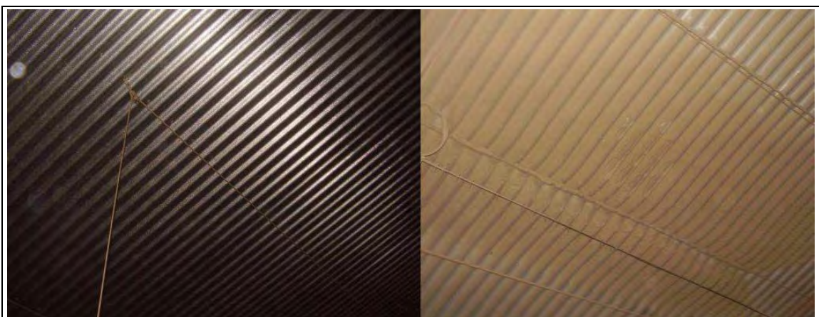
Figure 2.7: Effect of dust attraction caused by ionisation on the roof of a poultry shed
