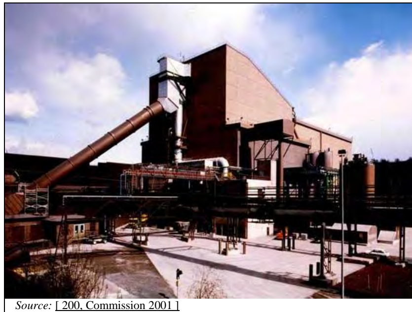
Figure 8.1: Electric arc furnace plant
