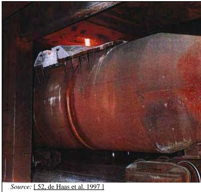
Figure 6.16: Charging of hot metal into torpedo ladle with dust suppression with inert gas
