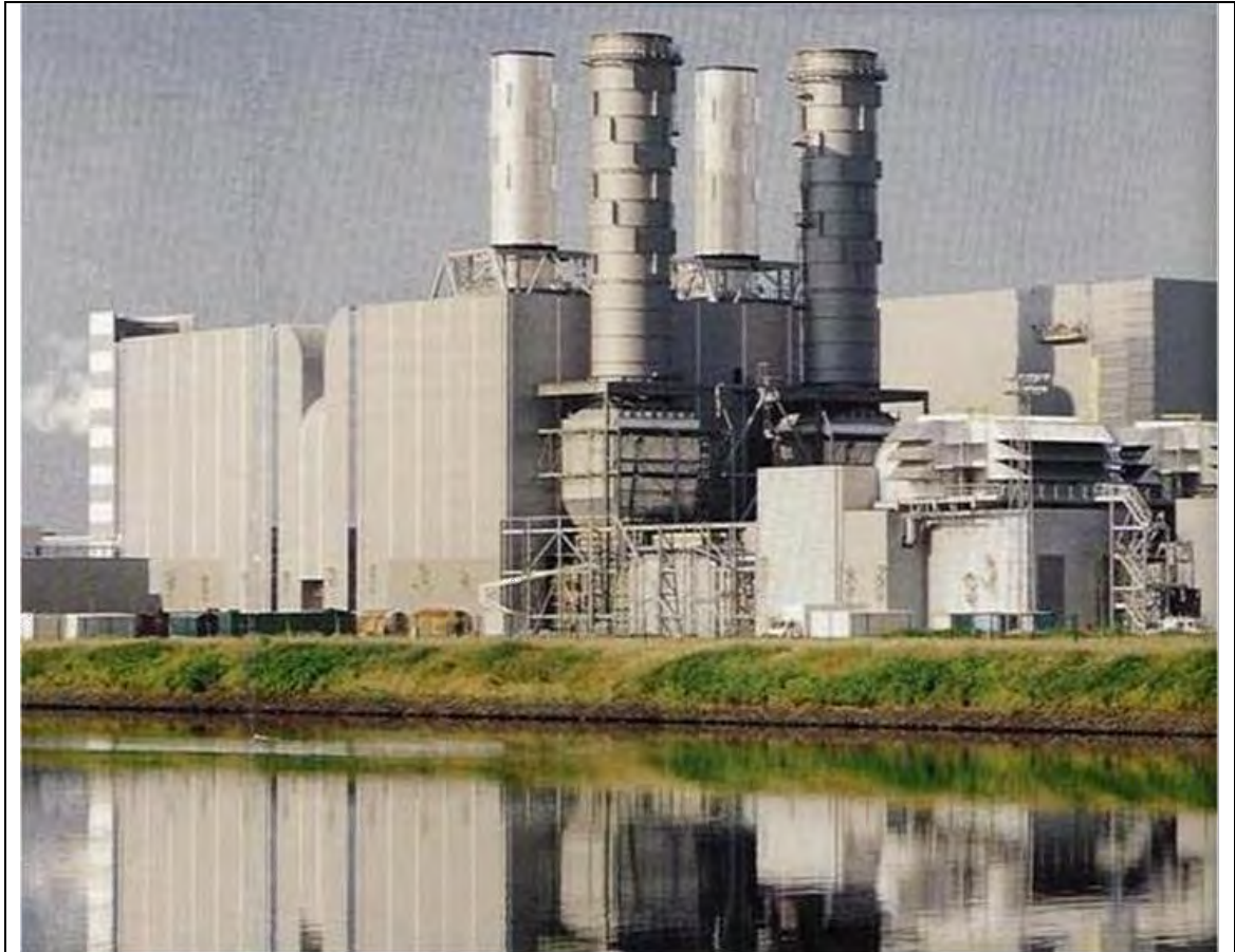
Figure 2.16: Recently built gas turbine combined cycle power plant in Belgium
