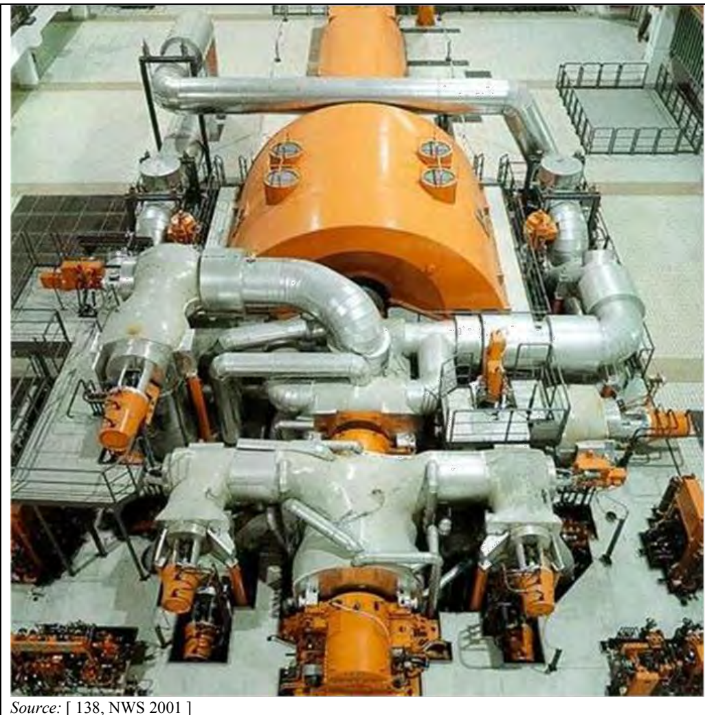
Figure 2.17: Steam turbine of a coal-fired power plant
