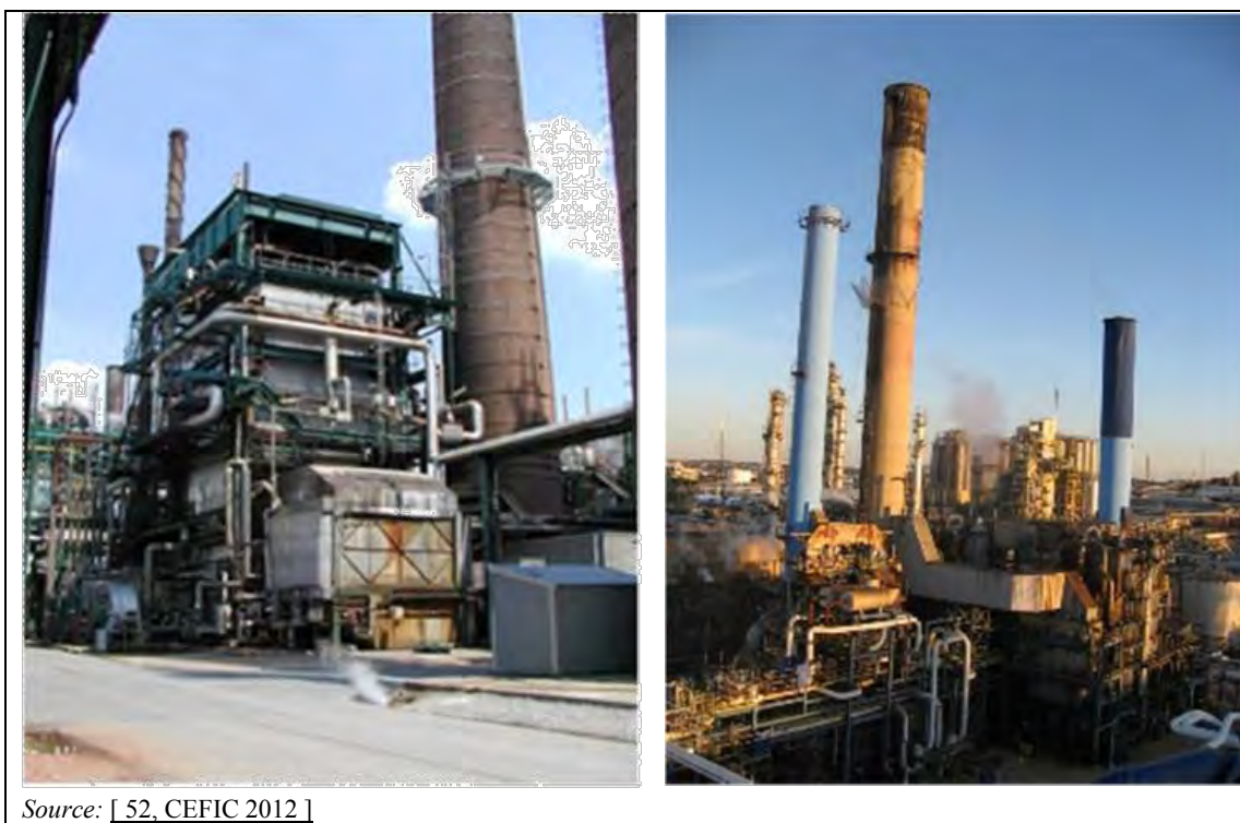
Figure 8.3: Utility boilers in chemical installations
