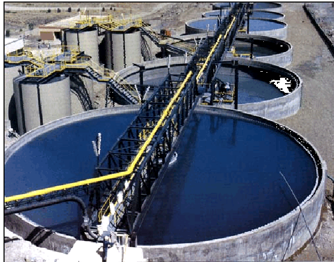
Figure 2.20: Continuous thickener
