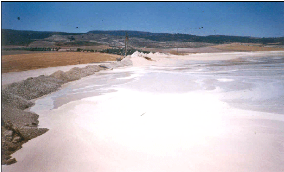
Figure 3.58: Old strontium TMF with tailings in structural zone [110, IGME, 2002]
