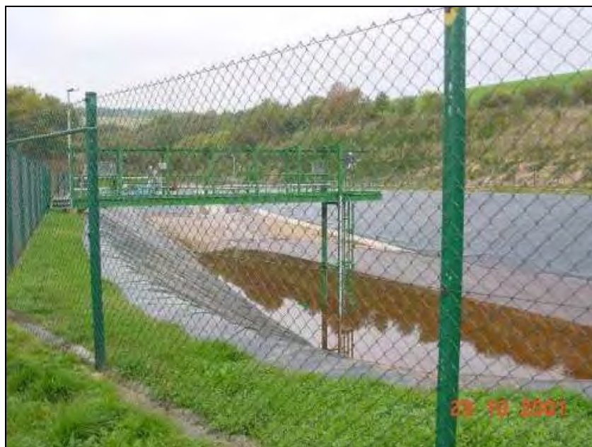
Figure 3.75: Water retention basin of German potash mine
