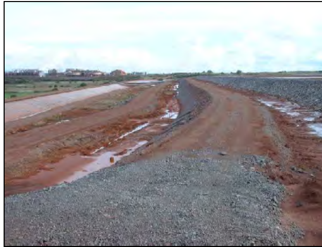
Figure 2.40: Dams raised using the upstream method at the Aughinish site
