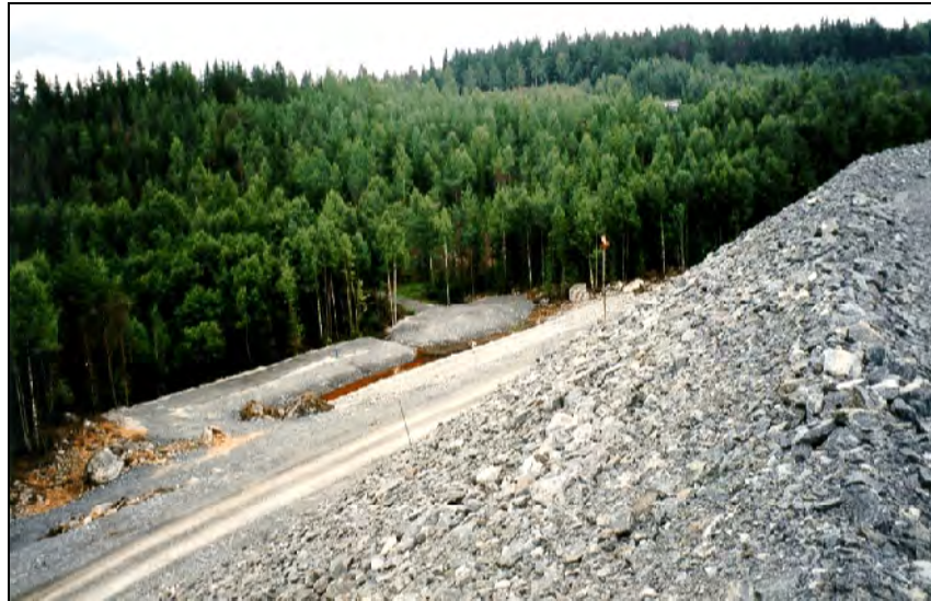
Figure 3.22: Ditch for collection and flow measuring of seepage water alongside the dam [66, Base metals group, 2002]
