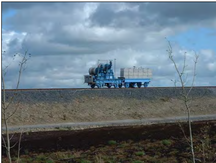
Figure 3.21: Electrically driven winch controlling the tailings distribution pipeline at the Lisheen TMF
