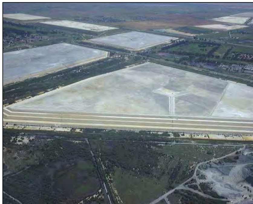
Figure 2.31: Tailings pond on flat land (Courtesy of AngloGold, South African Division)
