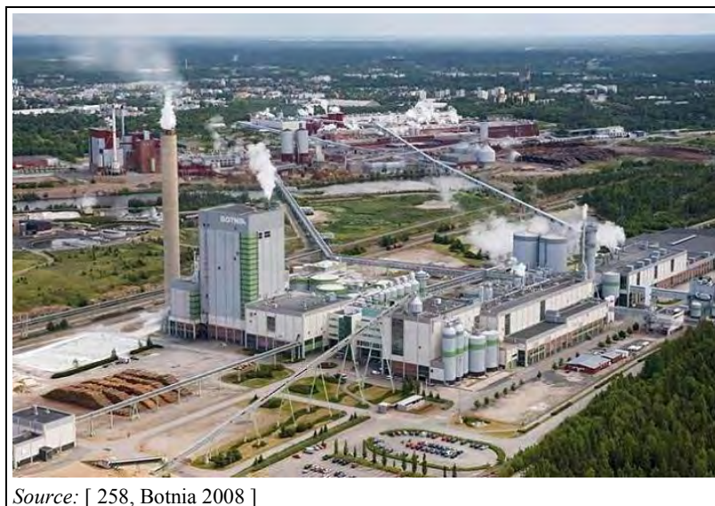
Figure 1.22: Aerial view of an integrated kraft pulp, mechanical pulp and paper site with a power plant and a waste water treatment plant
