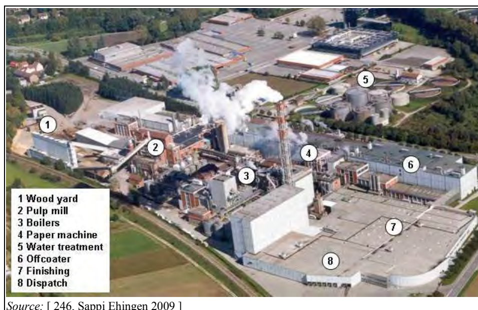
Figure 4.3: Aerial view of an integrated sulphite pulp mill producing coated fine paper including the power plant (centre) and the waste water treatment plant (back right)
