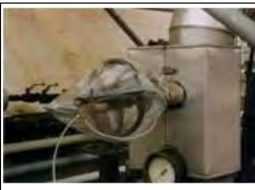
Figure 3.38: Bagging of a leaking valve
