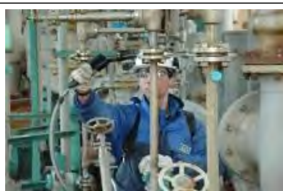
Figure 3.37: Leak concentration measurement
