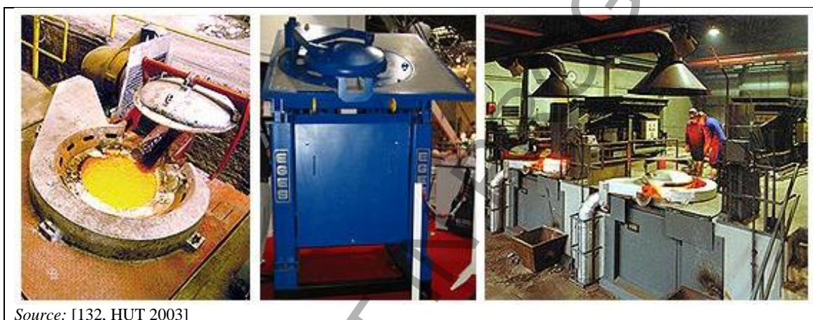
Figure 2.18: Coreless induction furnaces
