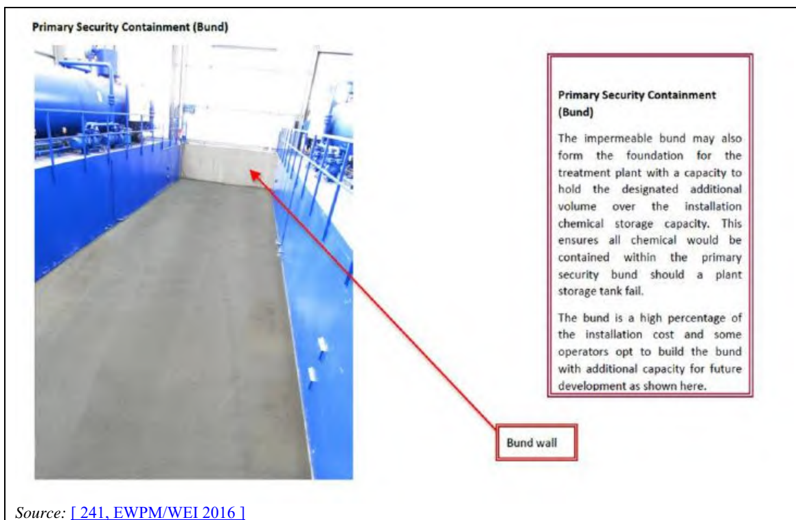
Figure 15.21: Design examples for process containment
