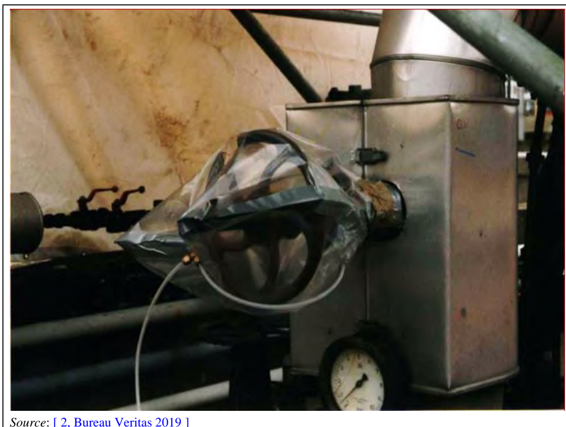
Figure 3.58: Bagging of a leaking valve
