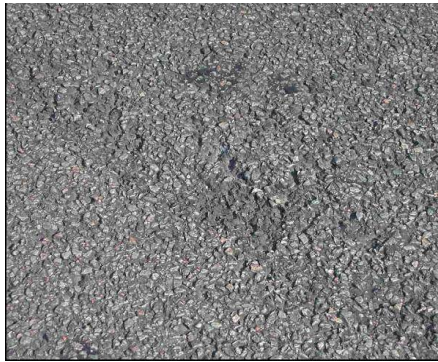
Figure C6 Ravelling and fretting
