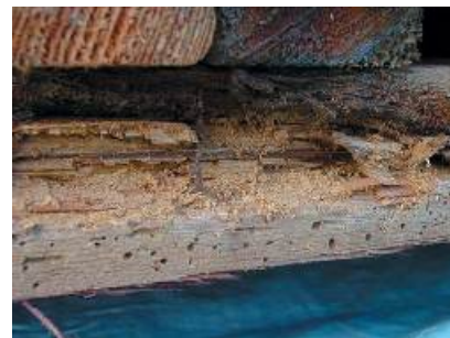
Figure 6.13 Wood frass from boring insect
